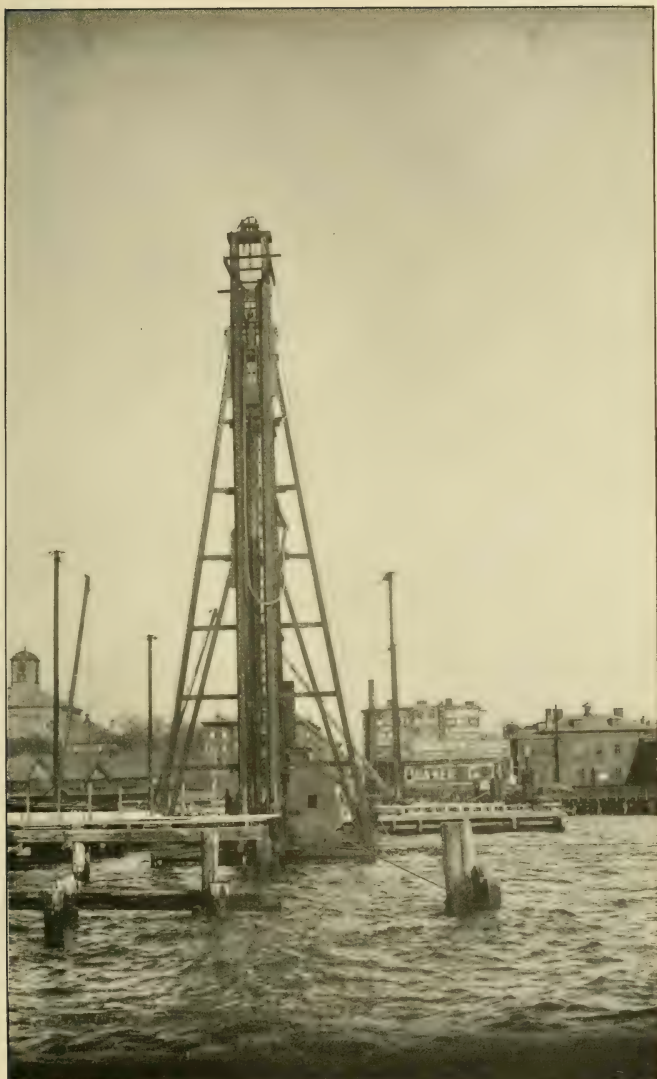
DRIVING OF FOUNDATION PILES. PILE IN POSITION READY TO DRIVE.
