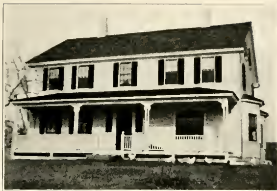
HOUSE IN WHICH I WAS MARRIED IN 1881. East Woodstock, Conn.
